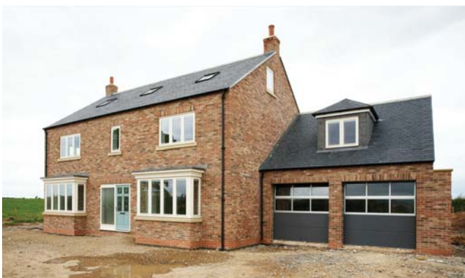
Project Name: Lowfields Farm, North Allerton
